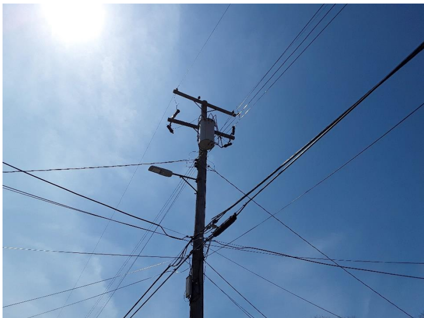
Pole-mounted electrical transformer located along an alley in the central-southern portion
