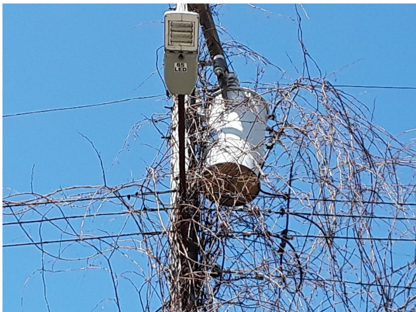
Typical pole-mounted electrical transformer
