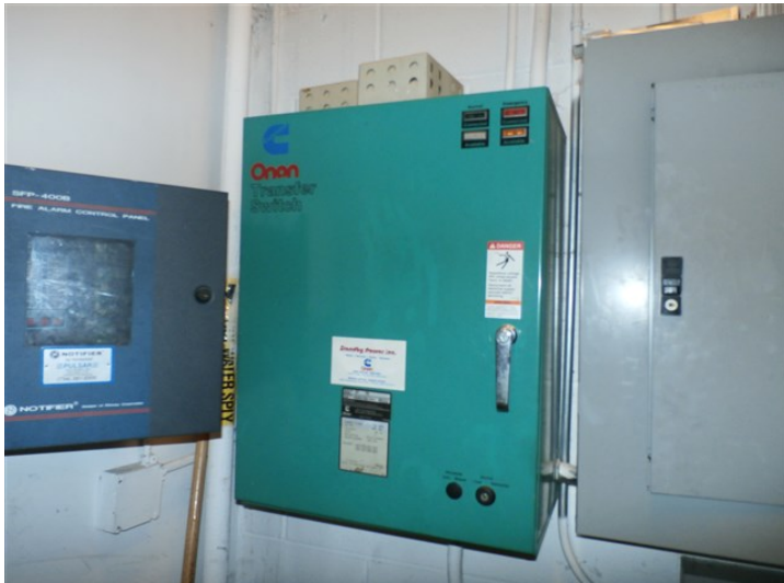
The fire alarm panel and generator transfer switch at the community building
