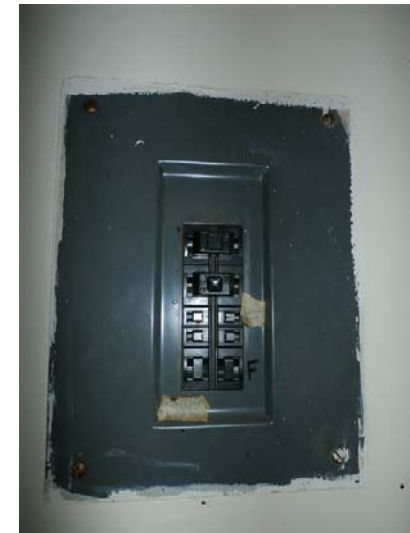
Typical unit circuit breaker panel with Stab-Lok breaker switches
