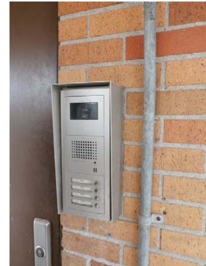
One of the walk up buildings' video intercom panels
