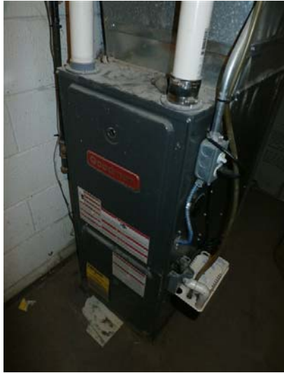
Typical unit Goodman warm air furnace
